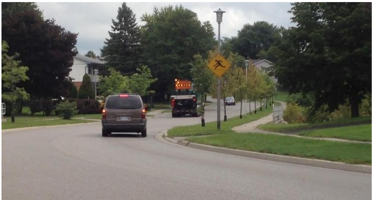
Figure 9: View of eastbound van and westbound car that must use the eastbound lane to pass the stopped work truck. Note that the van driver will ignore the warning sign indicating that he should pass the truck by steering around it to the left.
