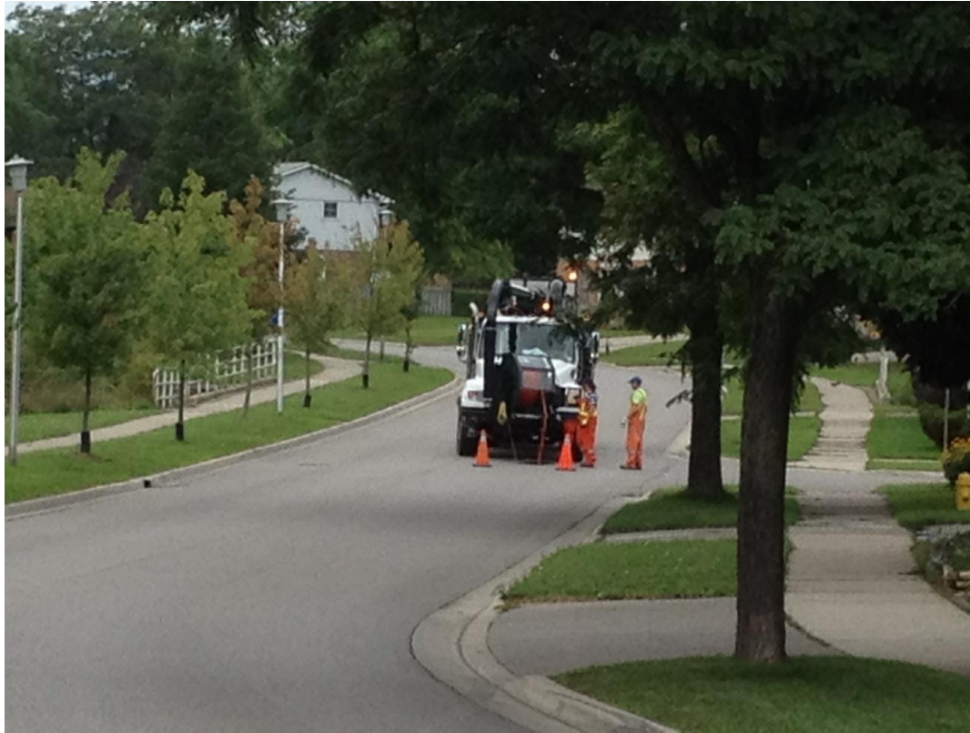
Figure 8: View, looking west, showing the work truck has blocked the westbound lane and there are no warning signs anywhere to warn drivers of its presence.
